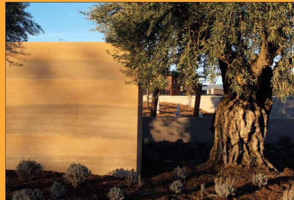
RAMMED EARTH WORKS COLLABORATED WITH CONTRACTORS CELLO & MAUDRU TO COMPRESS NATIVE AGGREGATES FROM NUN'S CANYON QUARRY INTO SIX STUNNING WALL PIECES SURROUNDING THE PROPERTY. PHOTO BY ASHLEY TEPLIN
